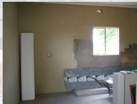
Building in progress
