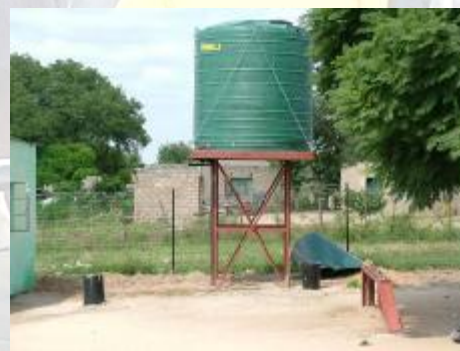
Water tank going up
