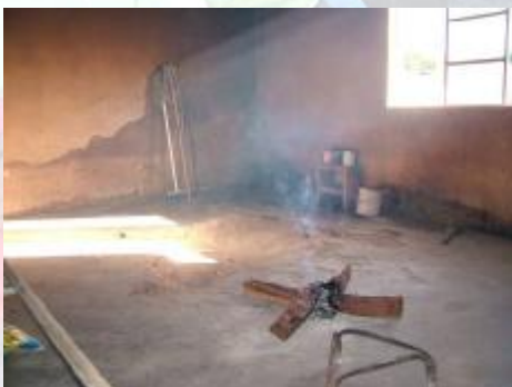
Old room we renovated for the new kitchen
